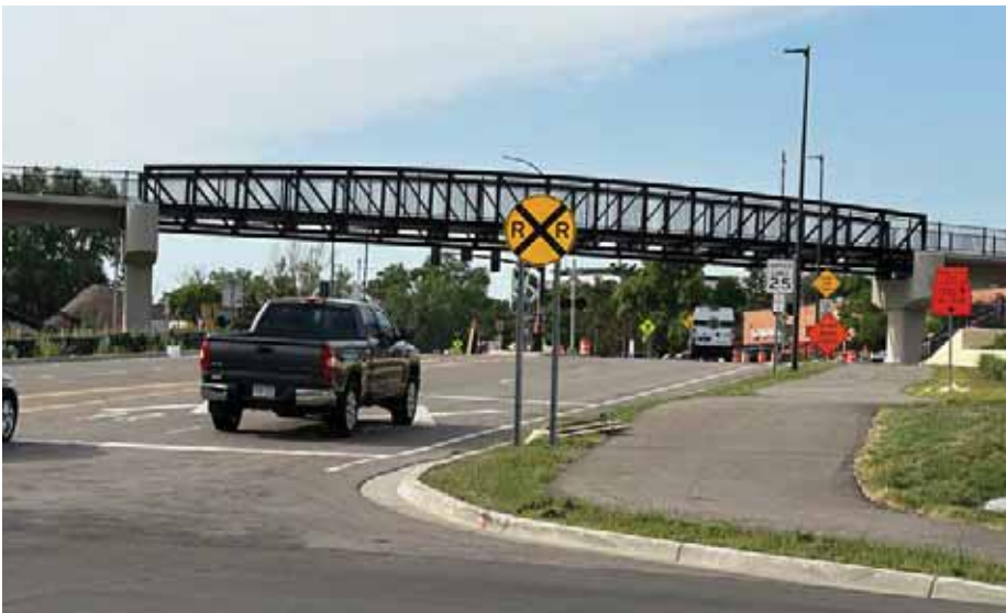
Highway 7 overpass in the Beltline Gateway
