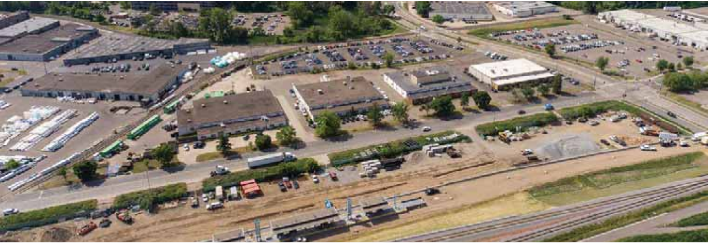
Existing Rail Spur
