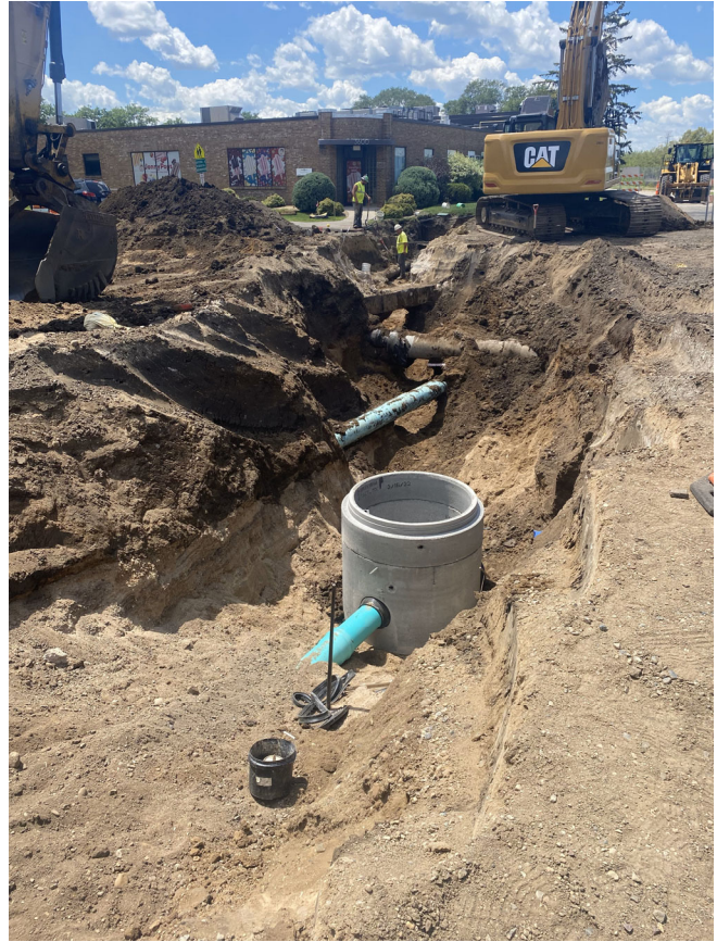
Underground utility construction
