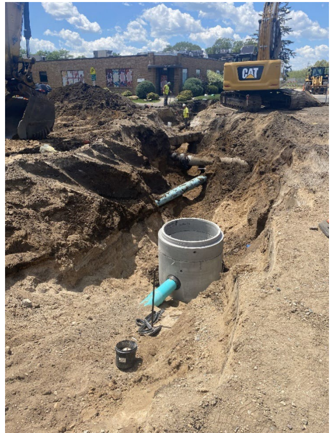
Underground utility construction
