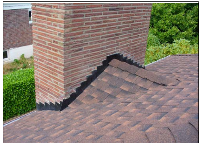
Cricket or saddle at chimney.
