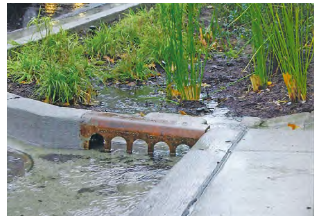
Flow-through curbs allow stormwater to be treated in specially designed treatment cells along streets.
