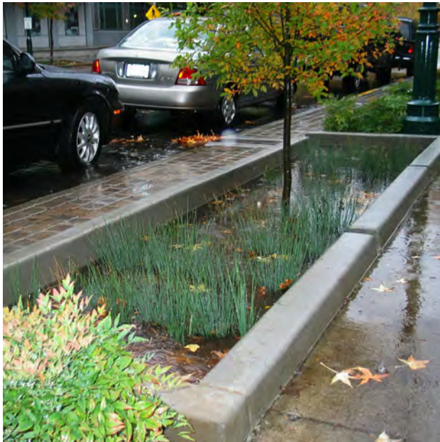
An interconnected system of stormwater treatment trenches should be developed to treat run-off from streets.
