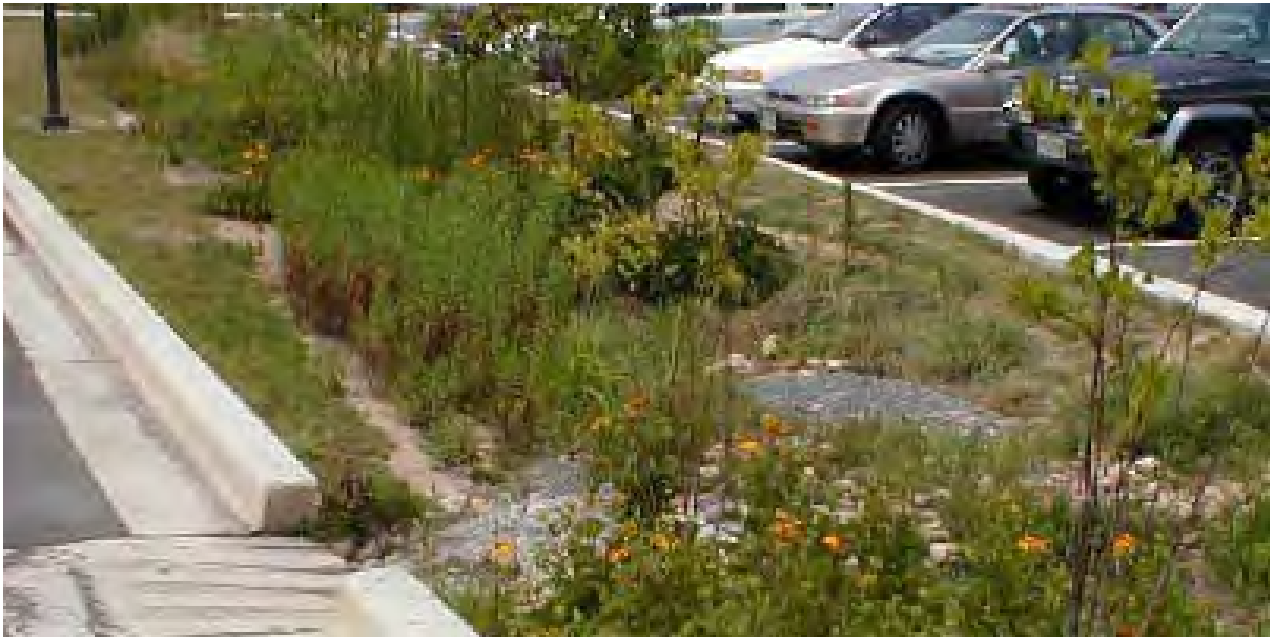
Curb cuts leading to rainwater gardens with native plant materials can be used to treat stormwater runoff from surface parking lots.
